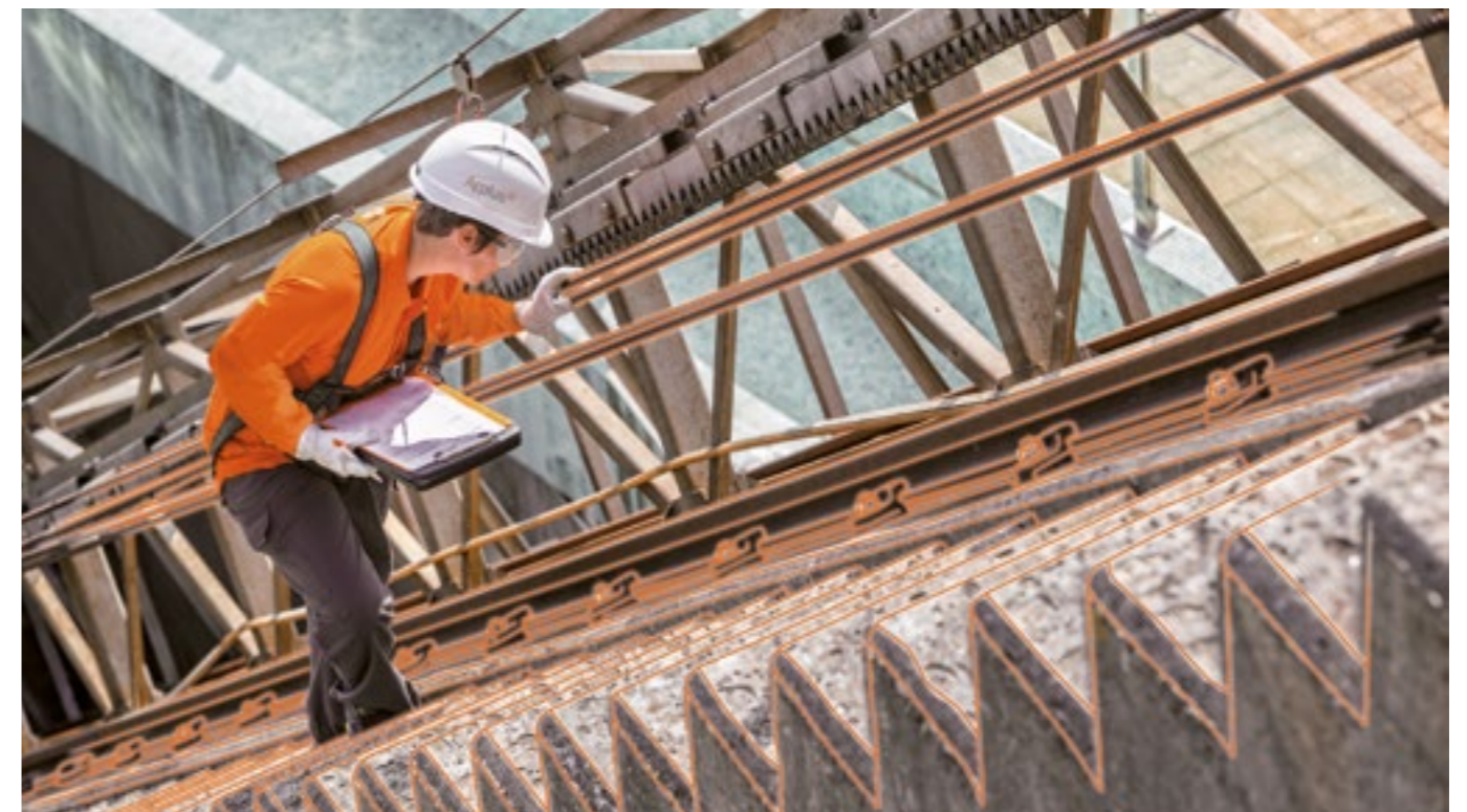
Statutory inspection in a cable car, Spain
