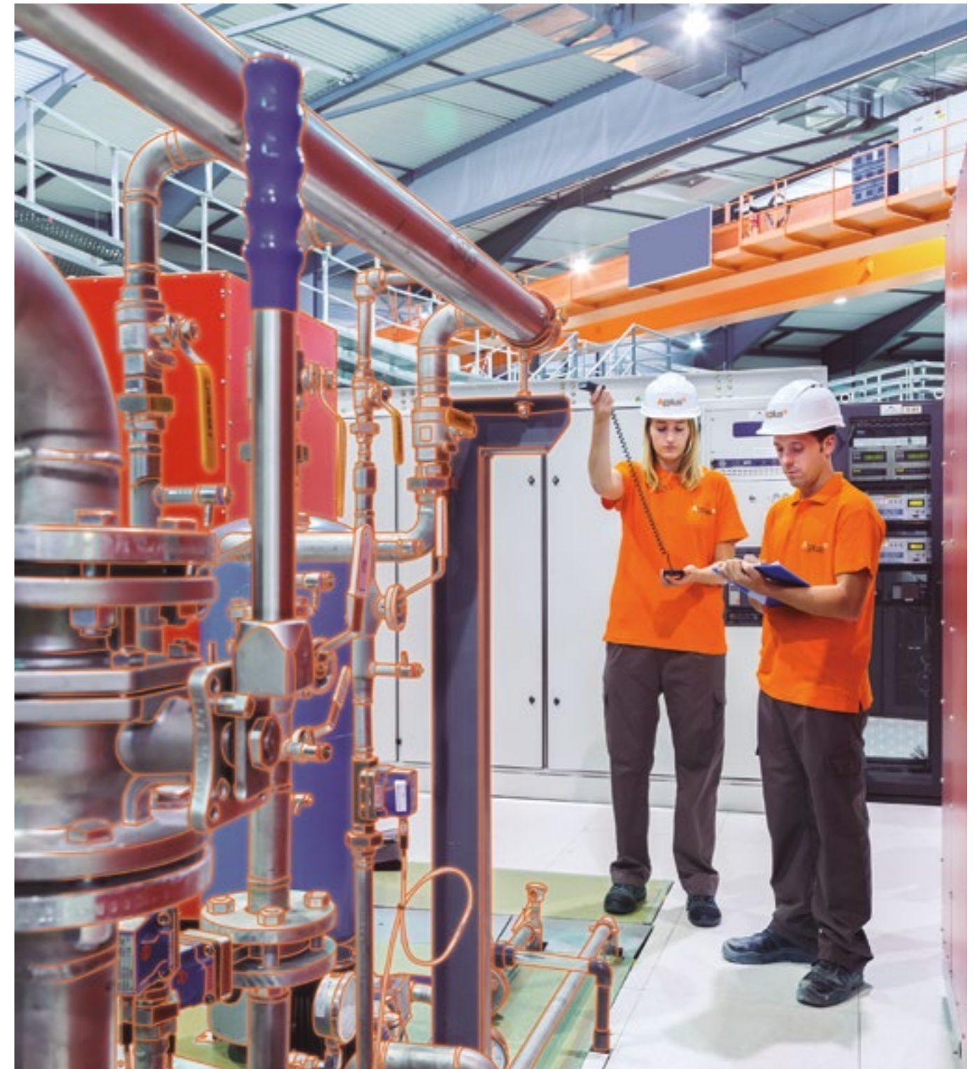
Quality control and technical assistance in building, Spain
