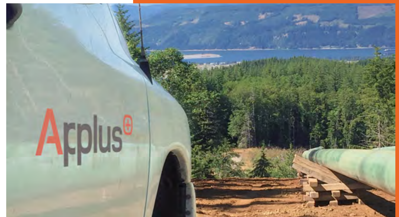
Pipeline integrity management
