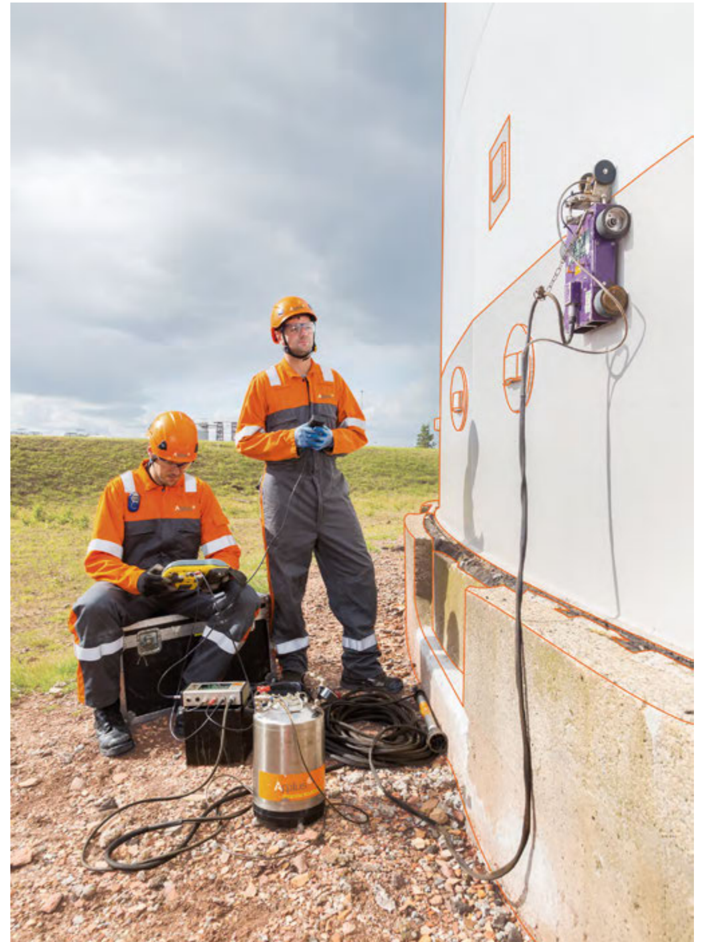
Non-destructive testing on a storage tank
