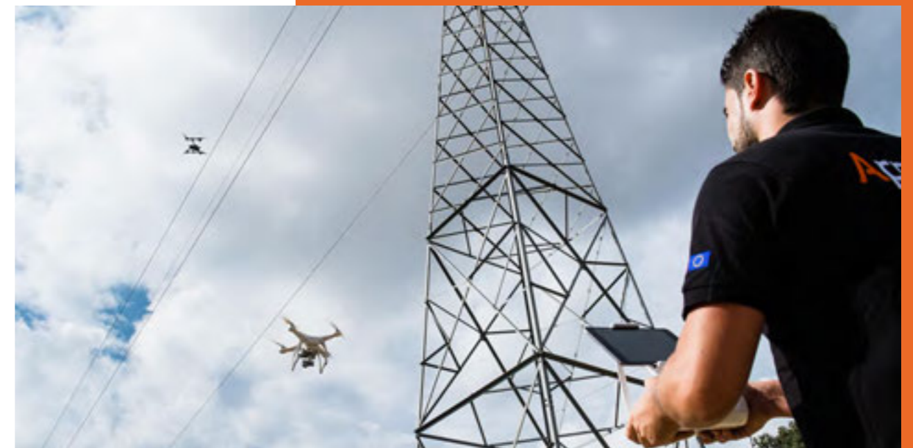
Drone inspection of power lines
